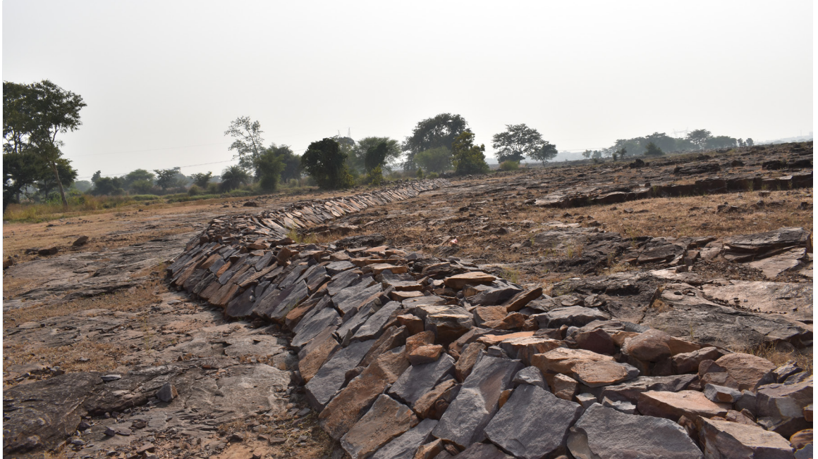
Contour bunding or embankment built in Barbaspur village, Chhattisgarh.
