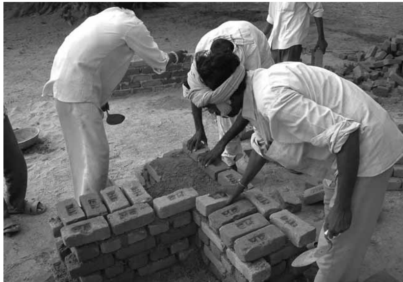
Masons certification programme in Datrana village, Patan District of Gujarat
