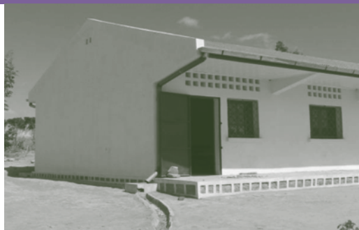
Primary school in Ambalamirary, Fianarantsoa Province. Building provided with gutters, downspouts, drop manhole and curved channel to evacuate rainwater from roof and surrounding area
